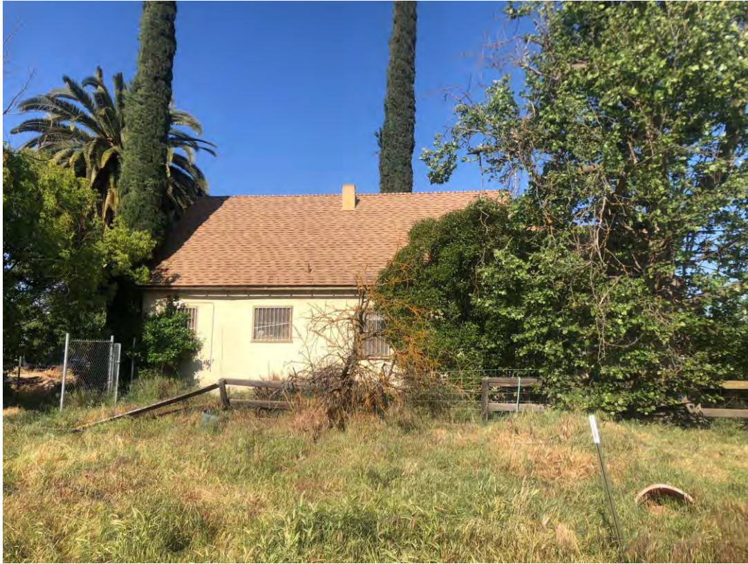
D) View looking west of the east facing facade. April 30, 2019. Acc. #201904fr2998
