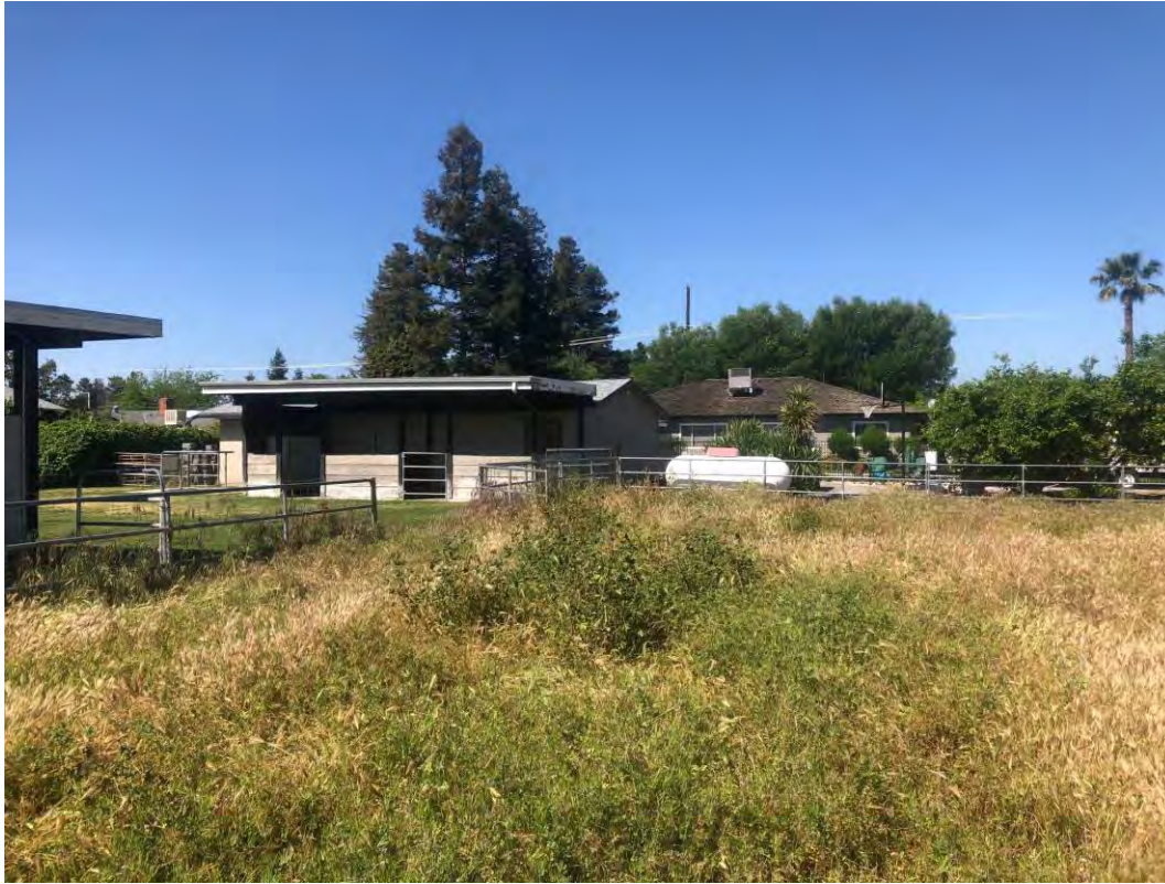
C) View looking northwest of the south and east facing facades of Outbuilding #1 April 30, 2019. Acc. #201904fr3021
