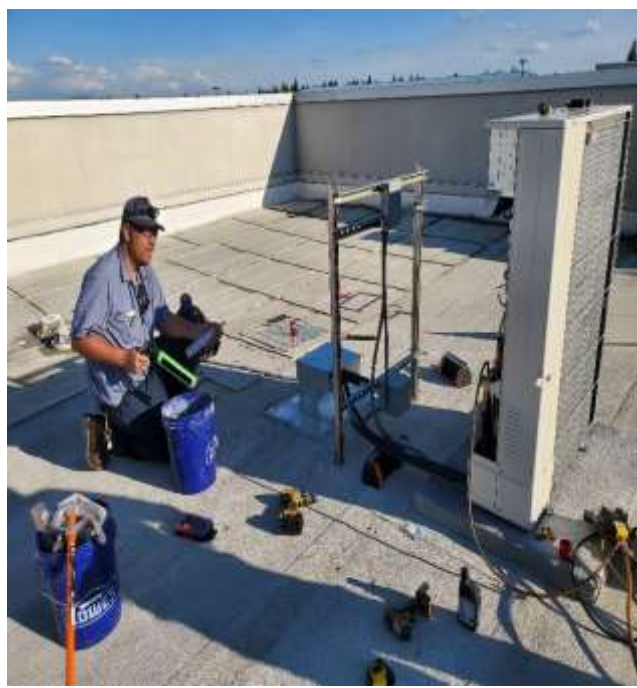
Facilities Maintenance Staff installed new mini split system at backup Police Dispatch.
