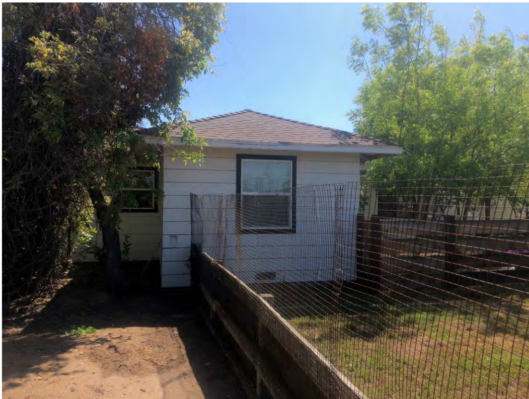
D) View looking southeast of the cross-gable section of the residence. April 30, 2019. Acc. #201904fr3015
