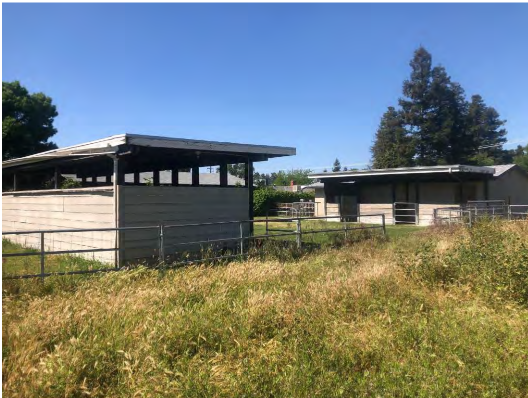
D) View looking northwest with Outbuilding #2 (left) and Outbuilding #1 (right). April 30, 2019. Acc. #201904fr3005
