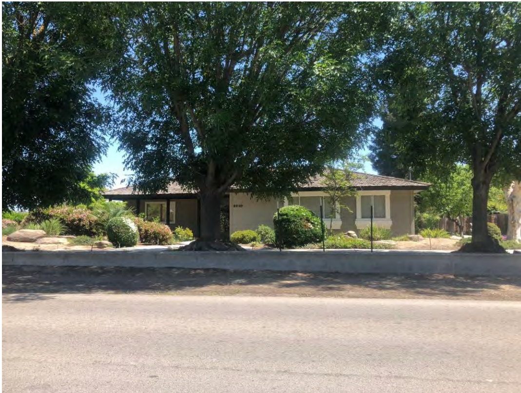
B) View looking east of the west facing facade of the residence. April 30, 2019. Acc. #201904fr3022
